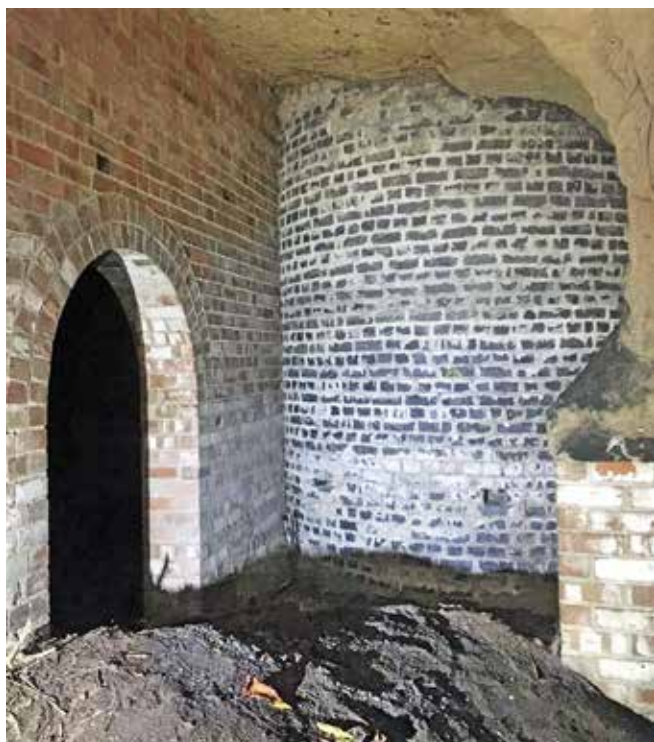
A former sand mine in private ownership showing Victorian industrial brick foundations for a house built above and later red-brick air-raid shelter reinforcement.
